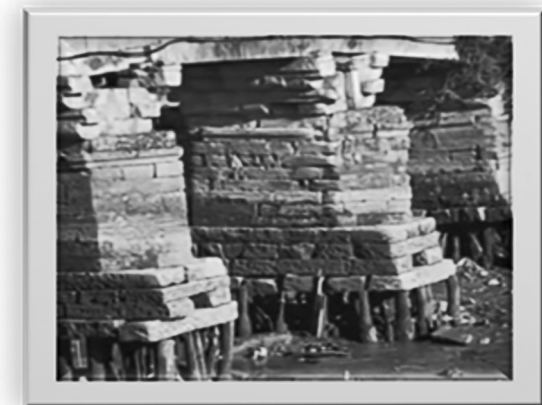
Fig. 1B: century old culvert is still standing on timber piling
