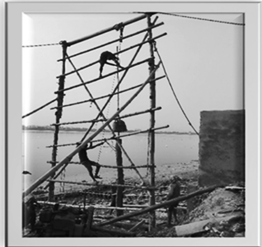
Fig. 1A: Timber Piling in progress at a Site
