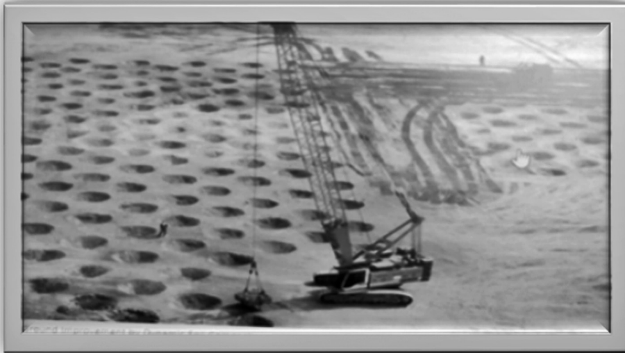
Fig. 6: An image of Dynamic Compaction
