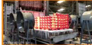
4 NOS (10 TON / 5 TON / 5TON / 1 TON) HEAT TREATMENT FURNACE WITH AUTO CONTROL WATER & AIR QUENCHING FACILITIES
